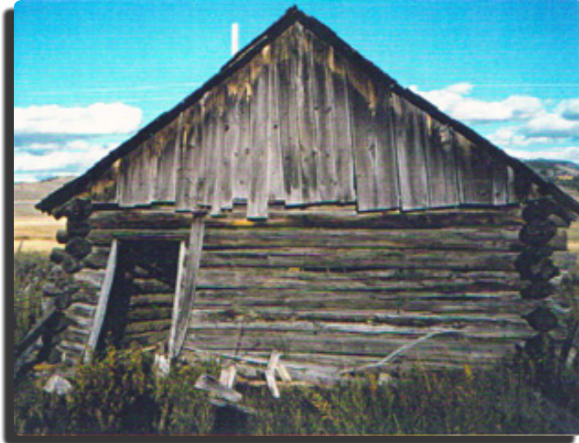
The actual dairy at the Lower Dairy in 1997. It sat over a natural spring where the cheese was made. By 2012, the roof of the dairy had collapsed.
