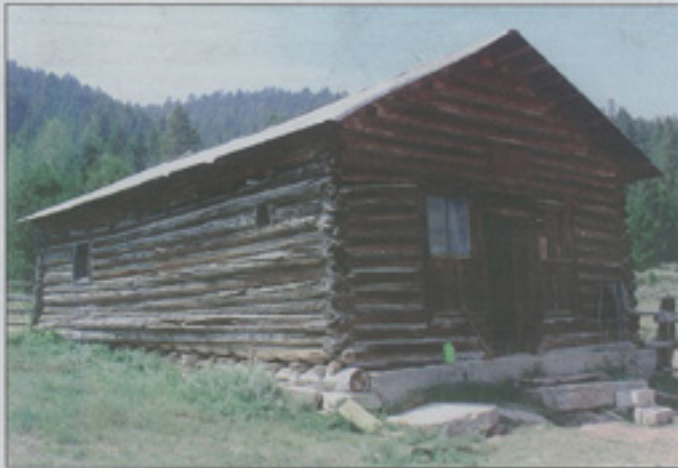
The drying room for cheese at the lower Williamsburg dairy is part of what is known to Star Valley residents as "The Dairies" west of Freedom. (Photo Courtesy of Denise Kunz)
