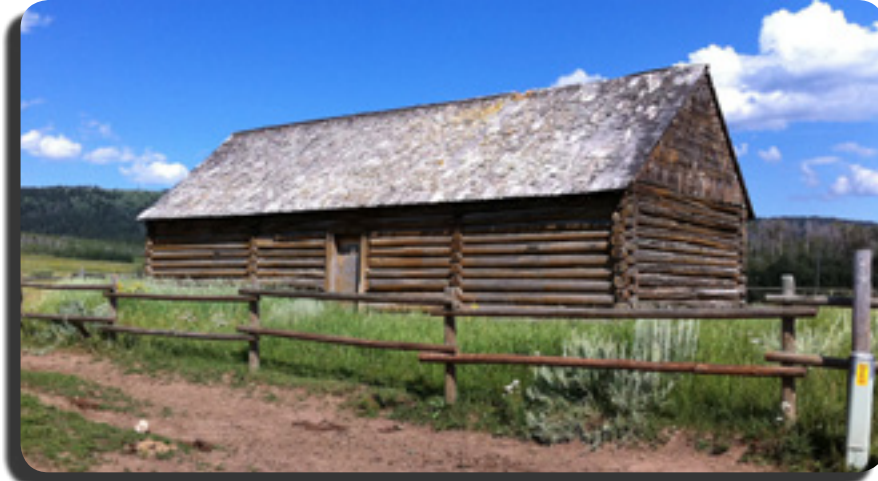
Above: East side of the Home of John Kunz III at the Upper Dairy
